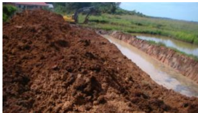
Leveling the excavated soil under the pond(final landscape)
